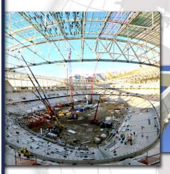
Overall, 110 tonnes of steel was rigged and welded on the project by a team of 36 qualified personnel – all successfully completed by Allweld, safely, within budget and on time.
