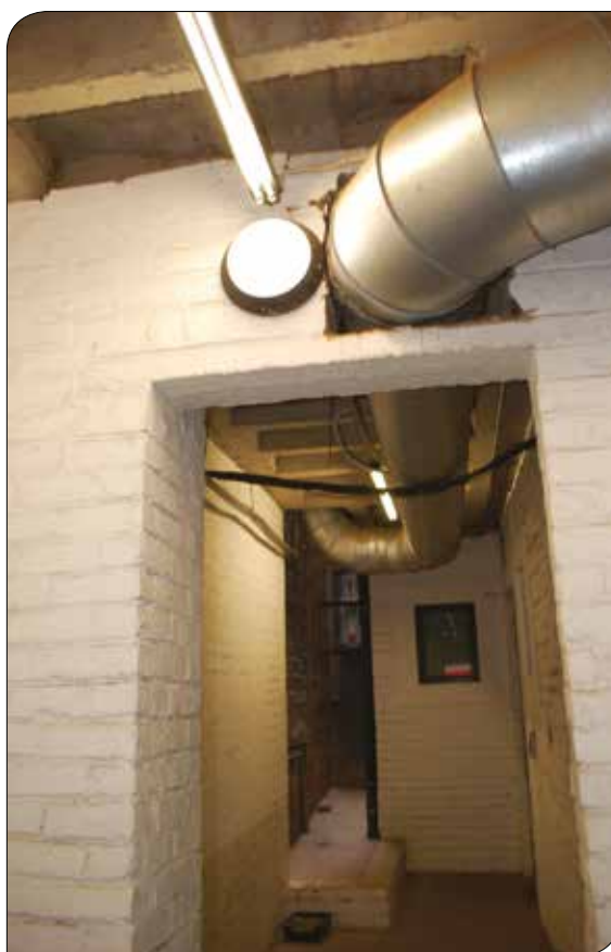
The ducting that distributes the ventilation throughout the building.
